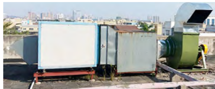
Replacement of the exhaust air ducts in the plug-in workshop
